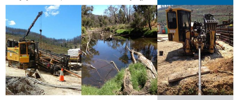
From the design pull-back calculations it was determined that a PN25 or SDR7.4 rated pipe would be required to meet the pull-back induced stresses. Through the DM Civil relationship with local pipe manufacturers, a special production run was able to be arranged for the higher than normal strength for this size of pipe. This allowed DM Civil to meet the construction programme set prior to several project unknowns being solved in the post-award design process.
