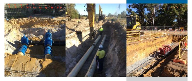
Buried existing services and overhead powerlines, stretching over 8.5km, were an issue. The project team spent a significant amount of time carefully locating, marking, pot holing and recording these services to guarantee there were no delays to the programme and to ensure everyone's safety.
