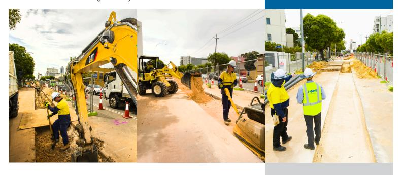
Part of the works required a 125mm Poly Pipe installation across Wellington Street into Outram Road. To minimise further disruption to traffic flows, DM Civil implemented HDD trenchless technology to complete this crossing. Through managing the drilling contractor and identifying the existing services in the vicinity of the drill shot in advance, this crossing was successfully completed with minimal effect on the local community.
