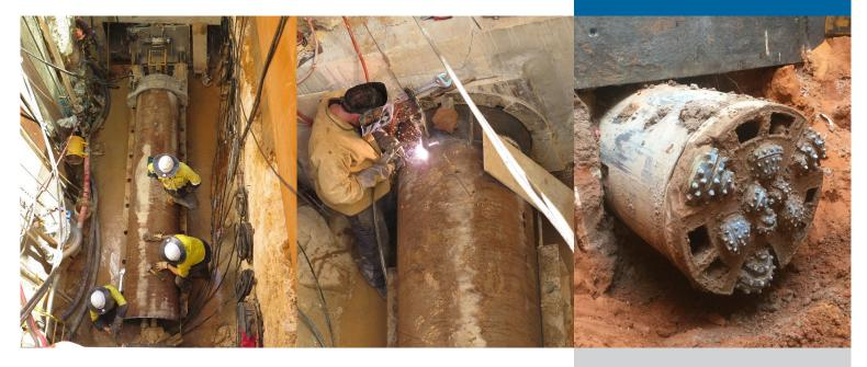
The systematic approach to tunnelling operations through internally developed procedures has allowed DM Civil to grow as a reliable tunnelling contractor. Critical aspects to the success of such a long drive include monitoring thrust forces, slurry flows, spoil volume (a method not widely used by others), drilling fluid properties and the use of additives and lubricants correctly matched to ground conditions. All of these elements ensure that thrust pressures remain within the allowable range.
