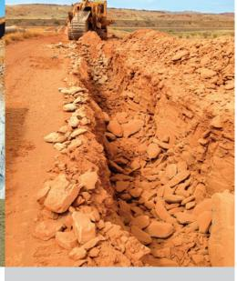
Amongst other material encountered, 'tuff' rock of variable weathering lay along the majority of the route. This area of the Pilbara contains the oldest and hardest rock on the planet. Additionally, the use of sand refill, paid on a provisional volume basis was kept to a minimum in the trencher sections.
