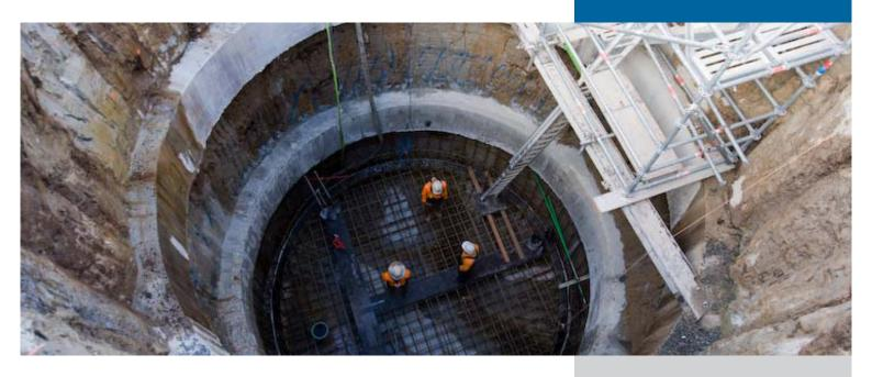
A primary focus of the works was minimising the disruption to surrounding residents. As the site was confined and had a high water table, conventional open excavation and dewatering methods were not viable. Our proposed alternative method used contiguous grout piles to create a sealed caisson from which we could excavate to the base of the pumping station with minimal requirement for dewatering and excavation. The contiguous piles also became the external formwork for the wet well.
