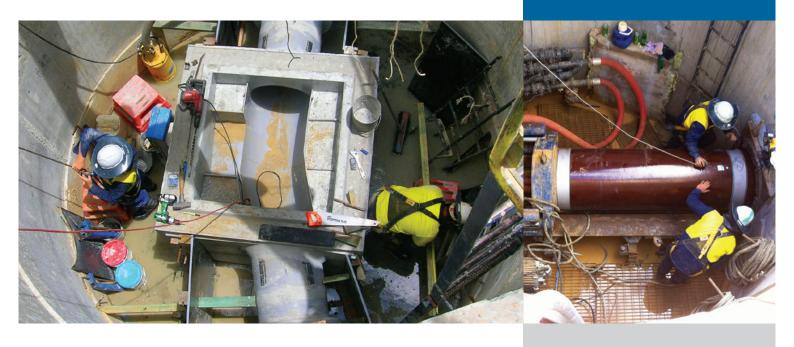
There were 2 sections to this project. The first involved the installation of 1,060m of DN600 vitrified clay jacking pipes constructed over 12 drives. The second involved the installation of 362m of DN500 vitrified clay jacking pipes over 5 drives. The entire service was installed successfully with a high degree of accuracy, given the significant number and length of drives necessary.
