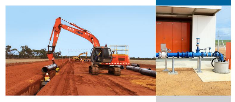
The majority of excavation along the alignment was completed using both of our Tesmec TRS 1475 and TRS 1300 Super trenching machines. The ground conditions in the area were mainly clay overlaying igneous and fractured rock. The trenching machines reduced the need for costly drill and blast operations and allowed the excavated material to be used for backfill along the alignment, significantly reducing the cost for the client.
