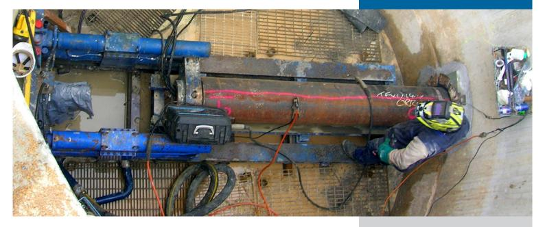
Trenchless technology drastically reduced the amount of dewatering required, which in turn allowed for Department of Water clearance for the project to proceed.
