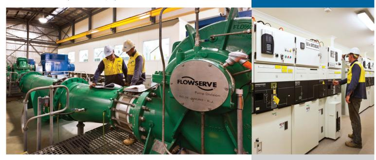
Walkaway is the largest water supply pumping station north of Perth. The building was complex in design with a roof structure that curved in both directions requiring innovation in manufacturing and construction techniques. Intricate concrete footing and slab details were constructed to suit several levels to support services and plant such as the pumps, control rooms and transformers.
