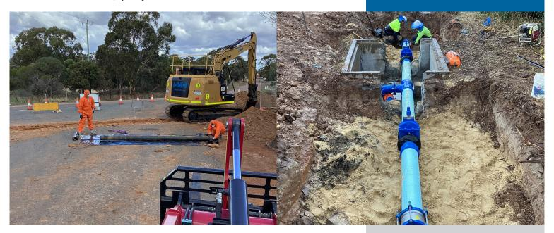
Cut-ins to the existing distribution main including demolition of the existing valve pit, installation of new valves, pipes, and an air valve had to be completed within an 8 hour shutdown period. DM Civil crews preplanned this shutdown sequence including the pre-assembly of all valves and pipe spools in time to minimise the scale and time of isolation related interruptions.
